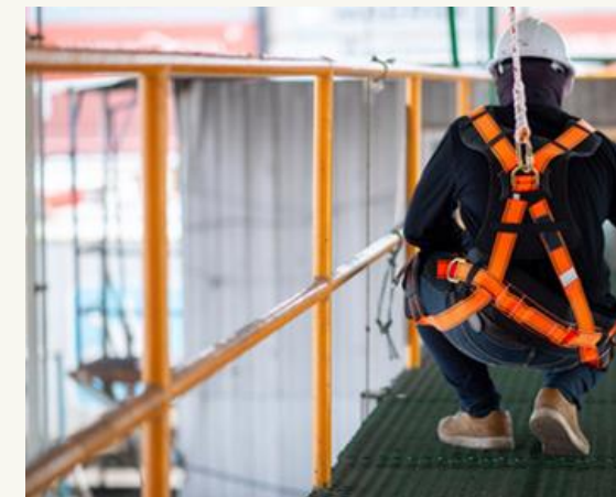
3. Pagar pengaman (Guard Railing)
