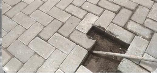
Bongkar Paving Block
